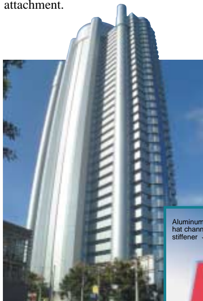
Plaza Centenário, Sao Paulo, Brazil Architect: Carlos Bratke, 1995 Aluminum stiffeners bonded to ACM panels.
